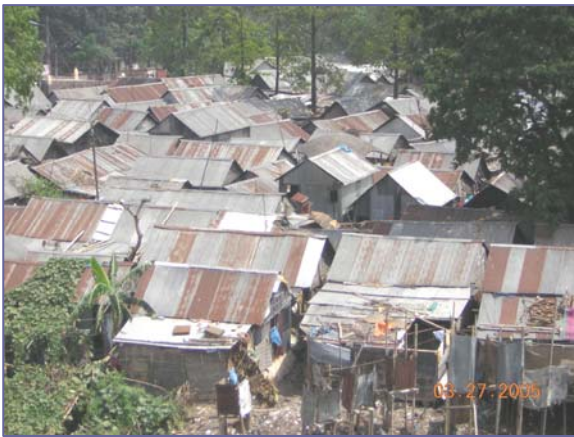
Photo - 3.24. Informal settlements in Dhaka City
